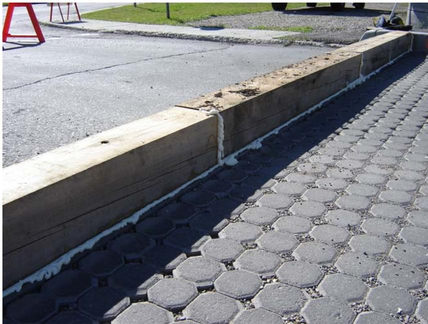
**Figure 3-21: Ponding Beam, Sealed with Polyurethane Expanding Foam**
