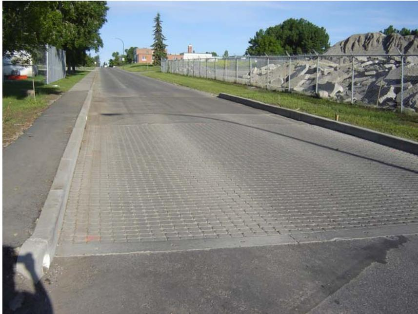
**Figure 3-1: Currie Barracks Permeable Pavement Installations (UNI Eco-Stone® in foreground, porous asphalt in background)**
