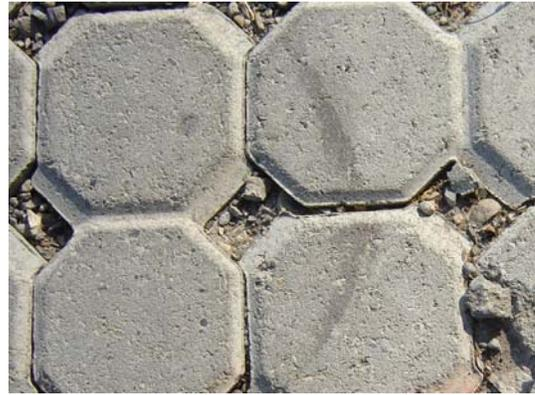
**Figure 4-12: Post-Maintenance Eco-Stone® , Infiltrator 'B' (Little Joint Fill Material Removed)**
