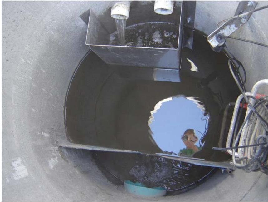
**Figure A-2: Weir in Manhole**
